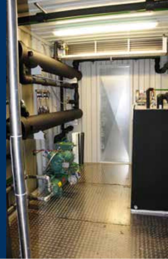
Ice water section of combined plants
