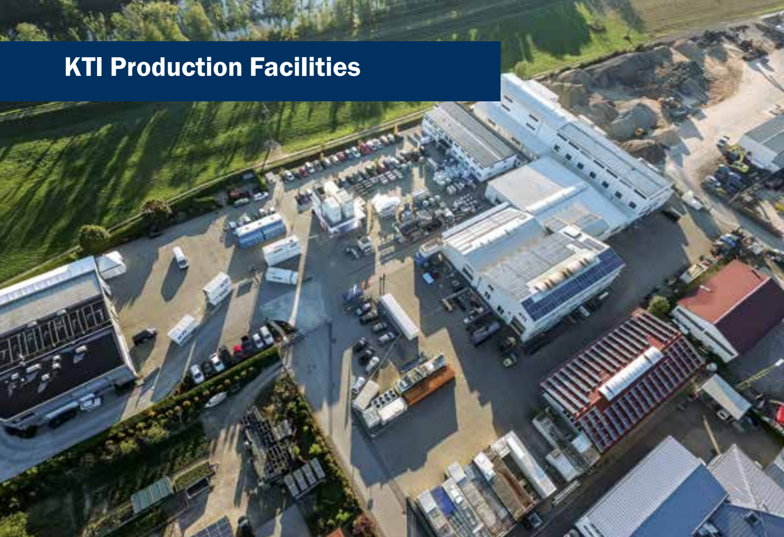
KTI Headquarter and Production Facility in Germany
