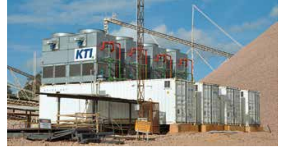
Water chiller systems CAC-w for aggregate cooling via wet belt systems
